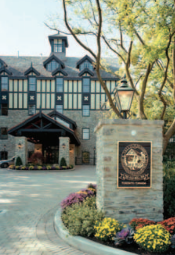
Old Mill Inn, Toronto, Canada
